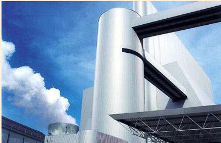
2 x 800 MW Lignite-Fired Power Plant Schwarze Pumpe, Germany
